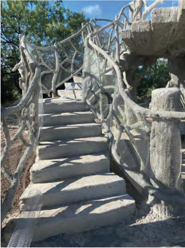
Pic #3 view of stairway with railing with mesh
