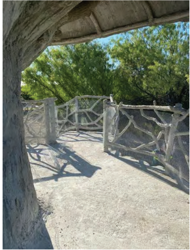
Pic #4 view of railing from upper deck
