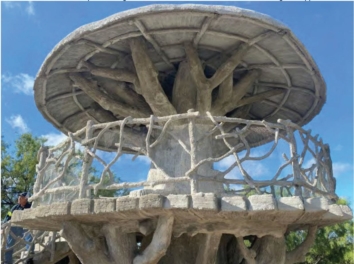
Pic #5 view of upper deck of tree with railing mesh installed
