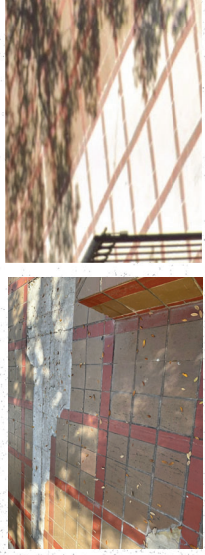
ALL THE EXTERIOR TILE NEEDS TO BE REMOVED AND REPLACED WITH THE NEW TILE SELECTION.
