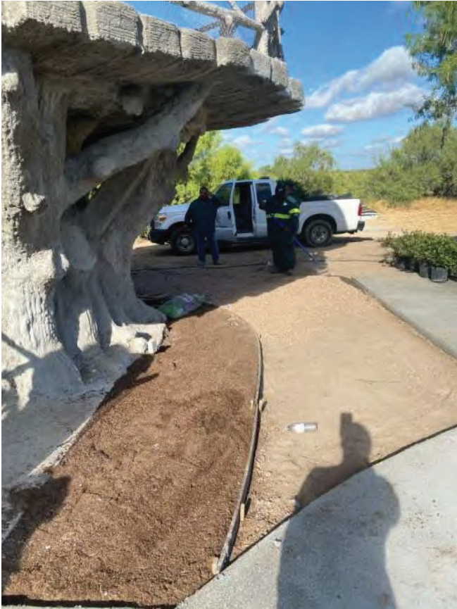
Pic #6 view of ongoing landscaping
