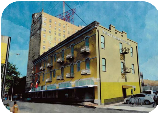
Southern Hotel Renovations
